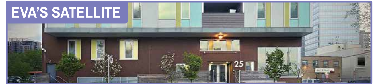
EVA'S SATELLITE Emergency shelter for 33 youth, with special health supports for substance use and mental health (Canada's first harm reduction shelter for youth).
